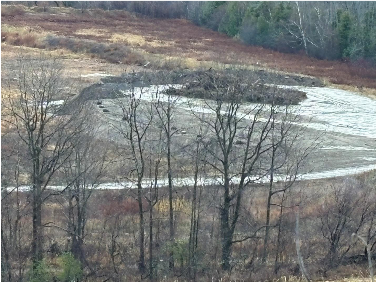
This picture shows the extensive build up of rubble, trees and brush to fill in the area where excavation of gravel went below the water table. This picture was taken November 22, 2024.
