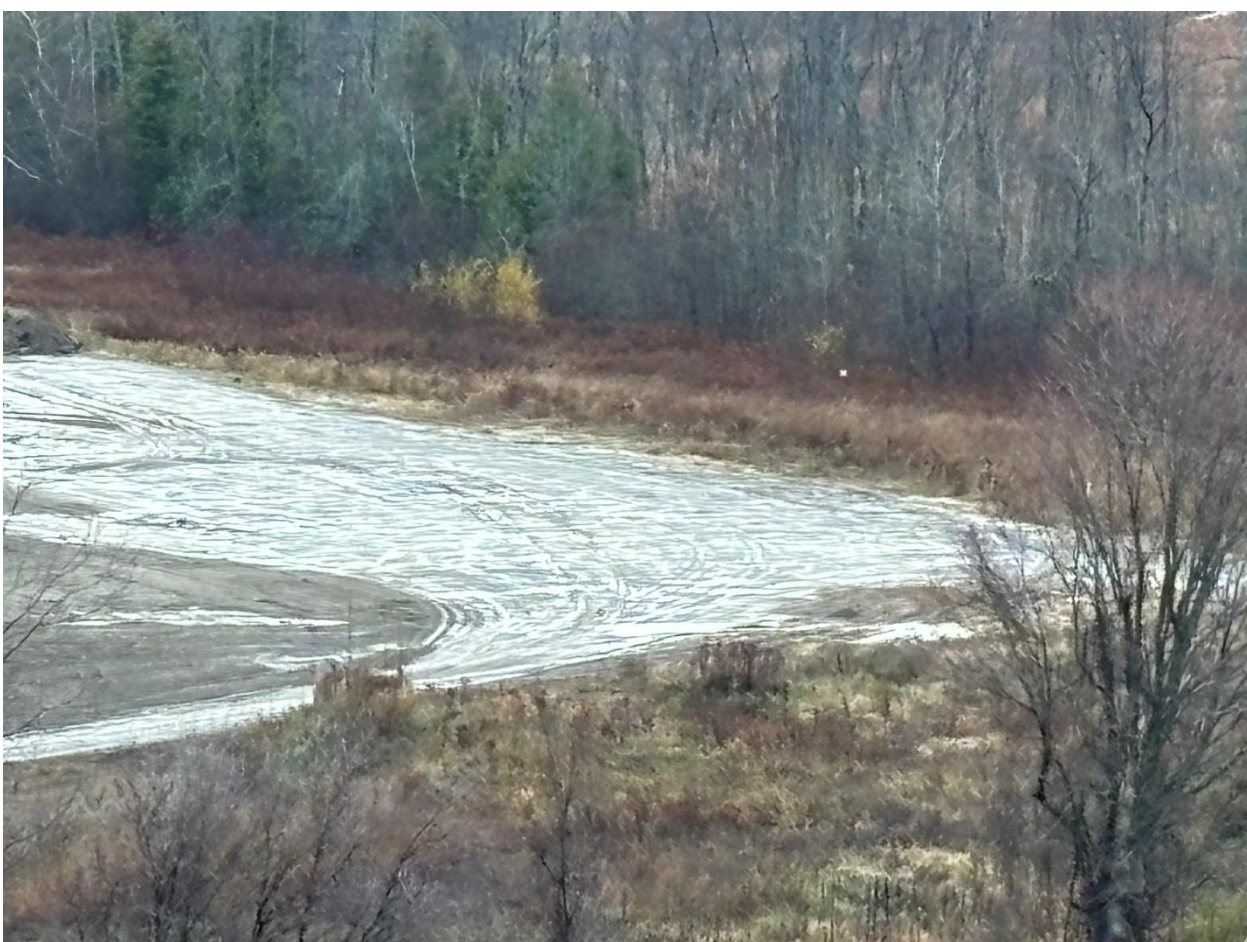
This picture shows the extensive build up of rubble, trees and brush to fill in the area where excavation of gravel went below the water table. This picture was taken November 22, 2024 following a light rain.
